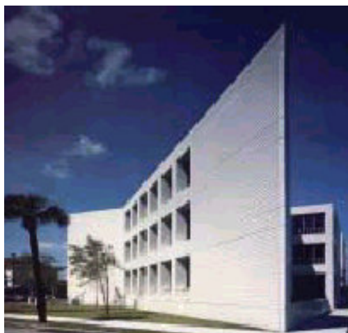
FIGURA 3.24- Commissioners of Republic WorksAdministrative Offices Charleston, South Carolina. (PCI, 1989, apud SILVA, 2002)
