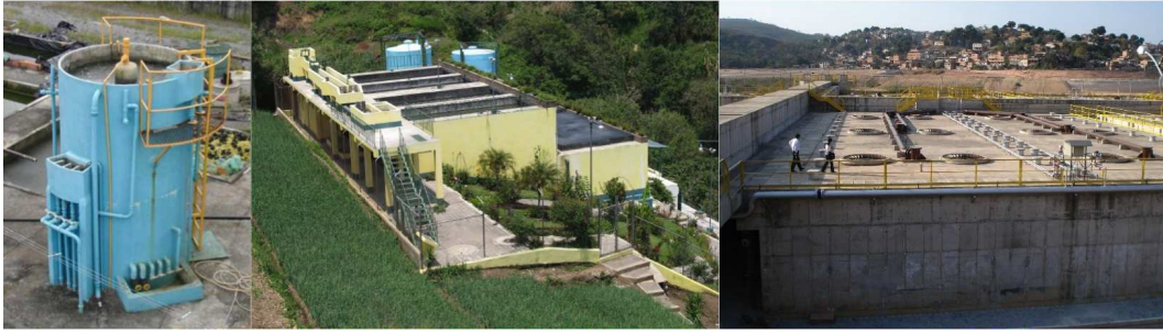
Figure 3. Upflow anaerobic sludge blanket (UASB) reactors used for different population ranges: left: hundreds of inhabitants (Belo Horizonte, Brazil, followed by maturation ponds); middle: thousands of inhabitants (Sololá, Guatemala, followed by a trickling filter with biogas storage tanks); right: one million inhabitants (Belo Horizonte, Brazil, also followed by trickling filters) (middle photo reproduced with permission of Stewart Oakley; left and right photos reproduced with permission of Marcos von Sperling).
