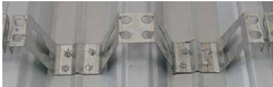
Figura 2.16 – Conector Stripcon 13
