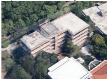
Figure 2: Analysed building under construction
