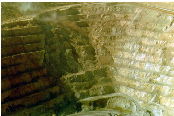
Figure 1: Mine slope failure (Hoek et al., 2000).
