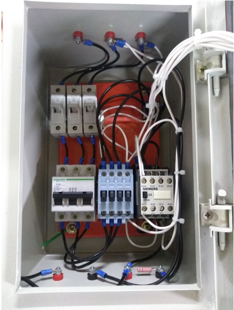
Figure A.3. Rectifying and protection box circuitry.
