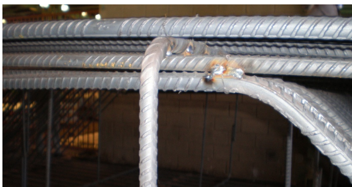
Figura 3.14 – Solda ponto (Ralf Schuttenberg, 2007)
