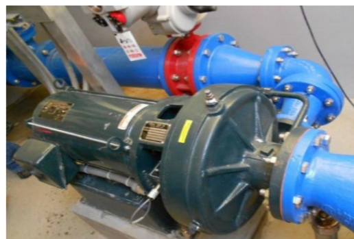
Figura 3.13 Turbina externa Rentricity flow to wire system.
