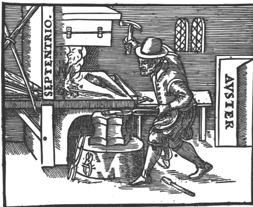
Figure 2 – A blacksmith forging a piece of cast iron for experiments with the magnet. The words avster and septentrio indicate the southern (= south) and northern (= north) polarities. Source: Gilbert 1600 , p. 139.
