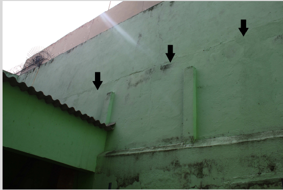
FIGURA 54 – [CHANFRO INADEQUADO]
