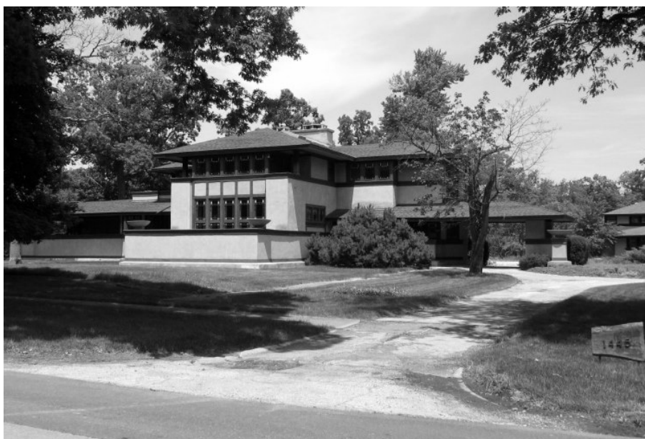
FIGURA 10 – Res. Ward-Willits, Highland Park, Illinois. Vista geral.
