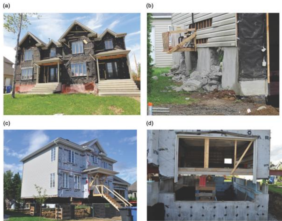
Figure 2. 8: Typical concrete foundation replacement process in the Trois-Rivières area: a) coating removal; b) foundation concrete demolition; c) shored house; and d) placement of the new concrete foundation (RODRIGUES et al. , 2016b)
