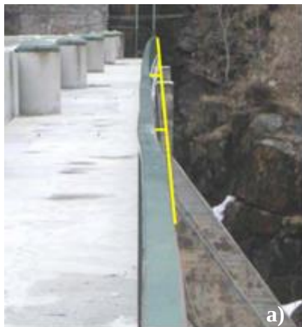
Figure 2. 3: Structural displacement at Graus dam (ARAÚJO, 2008 apud GOMIDES 2009)
