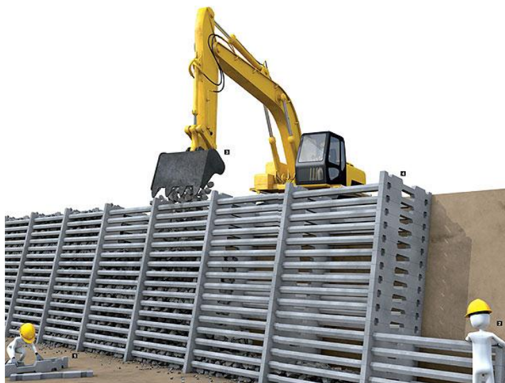
Figura 7: Muro de “Crib Wall”
