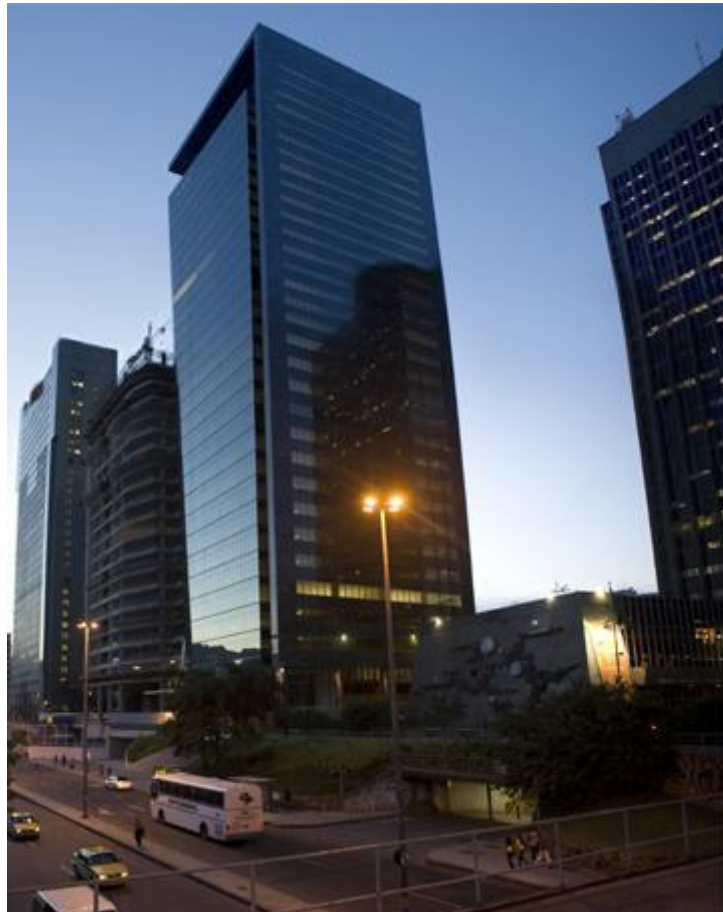
Figura 9. Ventura Corporate Towers – RJ
