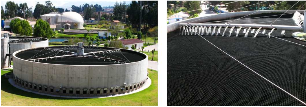
Figure 4. a) A plastic media trickling filter with a rotary hydraulic distribution arm designed for a flowrate of 40,000 m 3 /day (Cuzco, Peru). Note the ventilation ports around the base in the top photo. (b) close up of distribution system (photos by Stewart Oakley)
