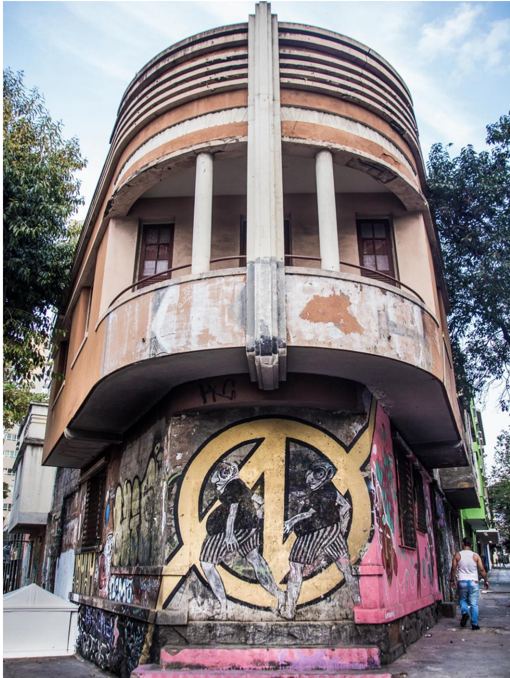
Facade. Photo by Cadu Passos, ceded by Kasa Invisível .
