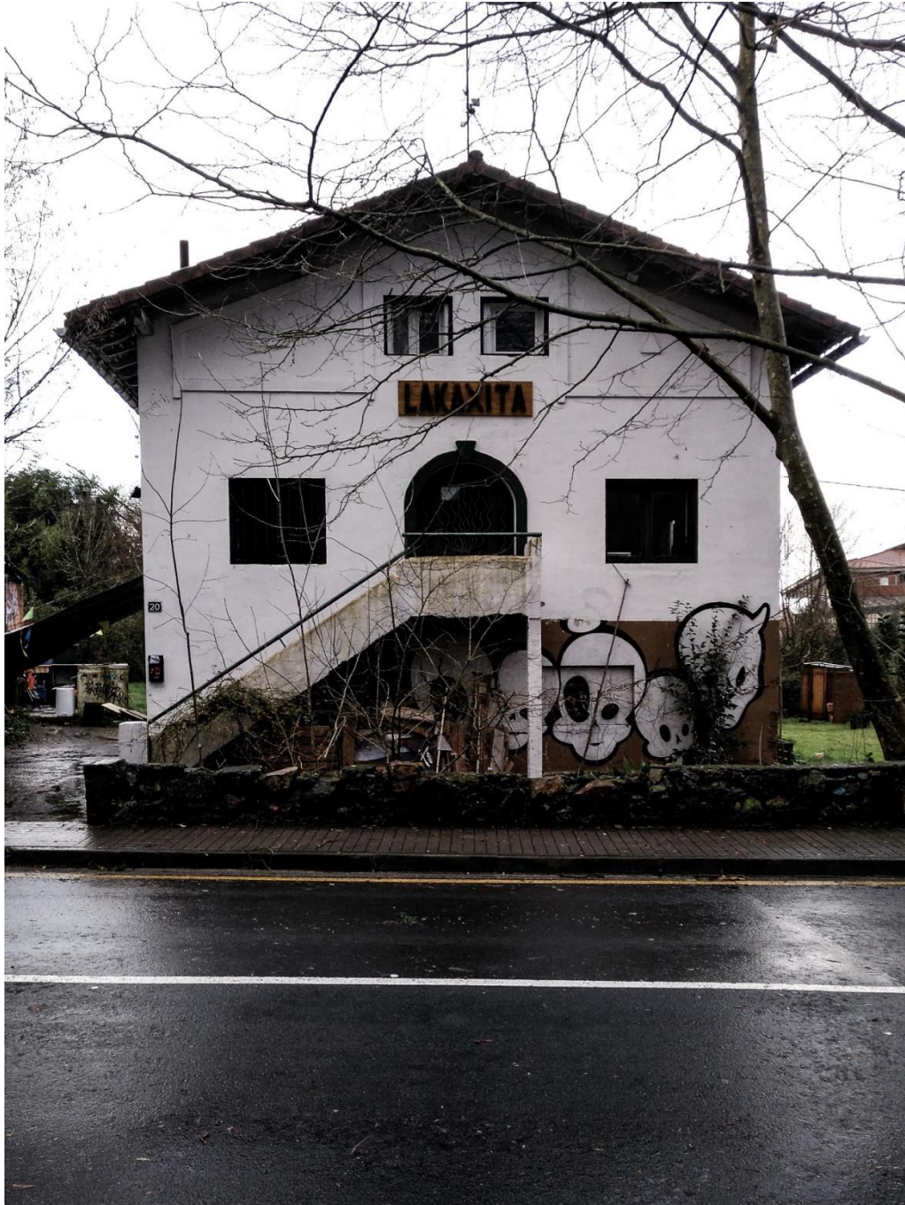
Facade. Photo by the author
