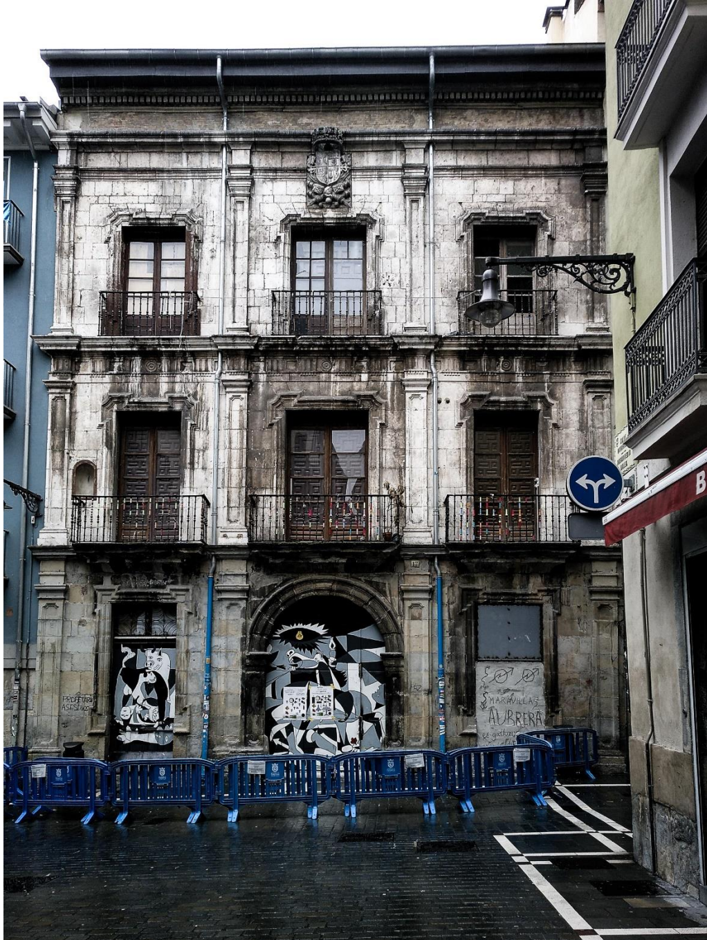
Facade. Photo by the author
