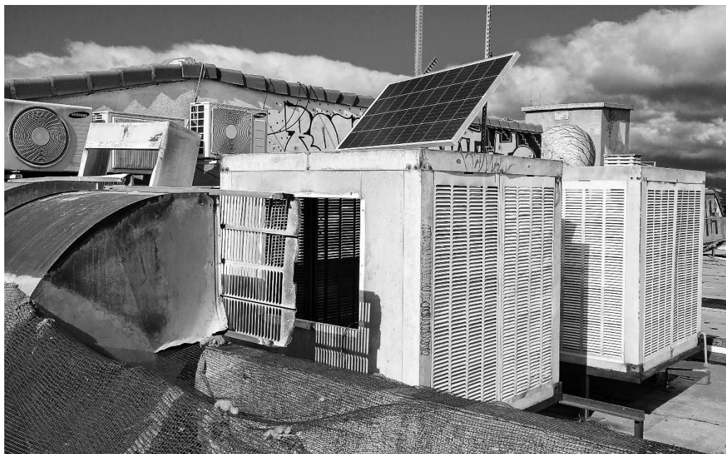
A) Side facade. B) Solar plate. Photos by the author
