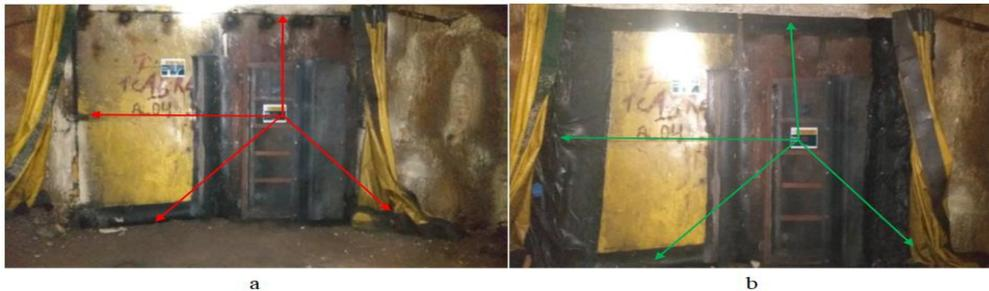
Figure 11- (a) air losses between doors; (b) application of seal on access doors to reduce air leaks.
