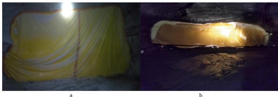
Figure 12- (a) unsealed curtains on the sides of the gallery; (b) curtains with seal on the edges of the gallery.
