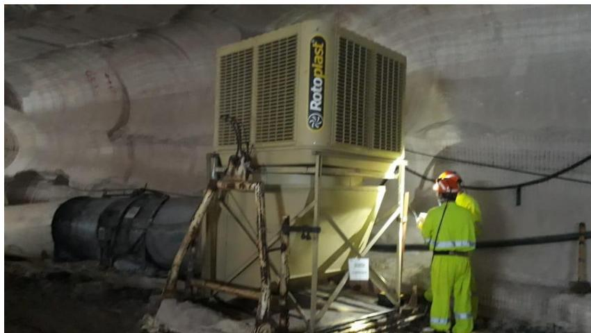
Figure 7- Installation of the air conditioner attached to the secondary fan.
