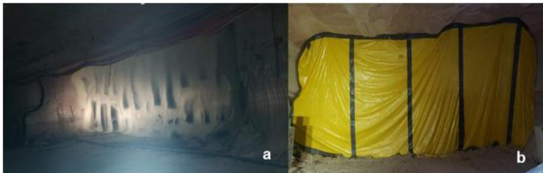
Figure 9- (a) belt siding sealed with polyurethane, (b) unsealed canvas siding.
