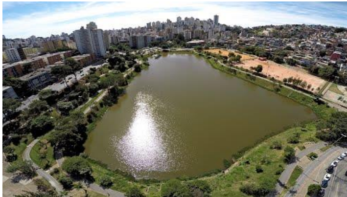
S3.16 Figure: Santa Lúcia dam in Belo Horizonte, Minas Gerais, Brazil (source: Internet).
