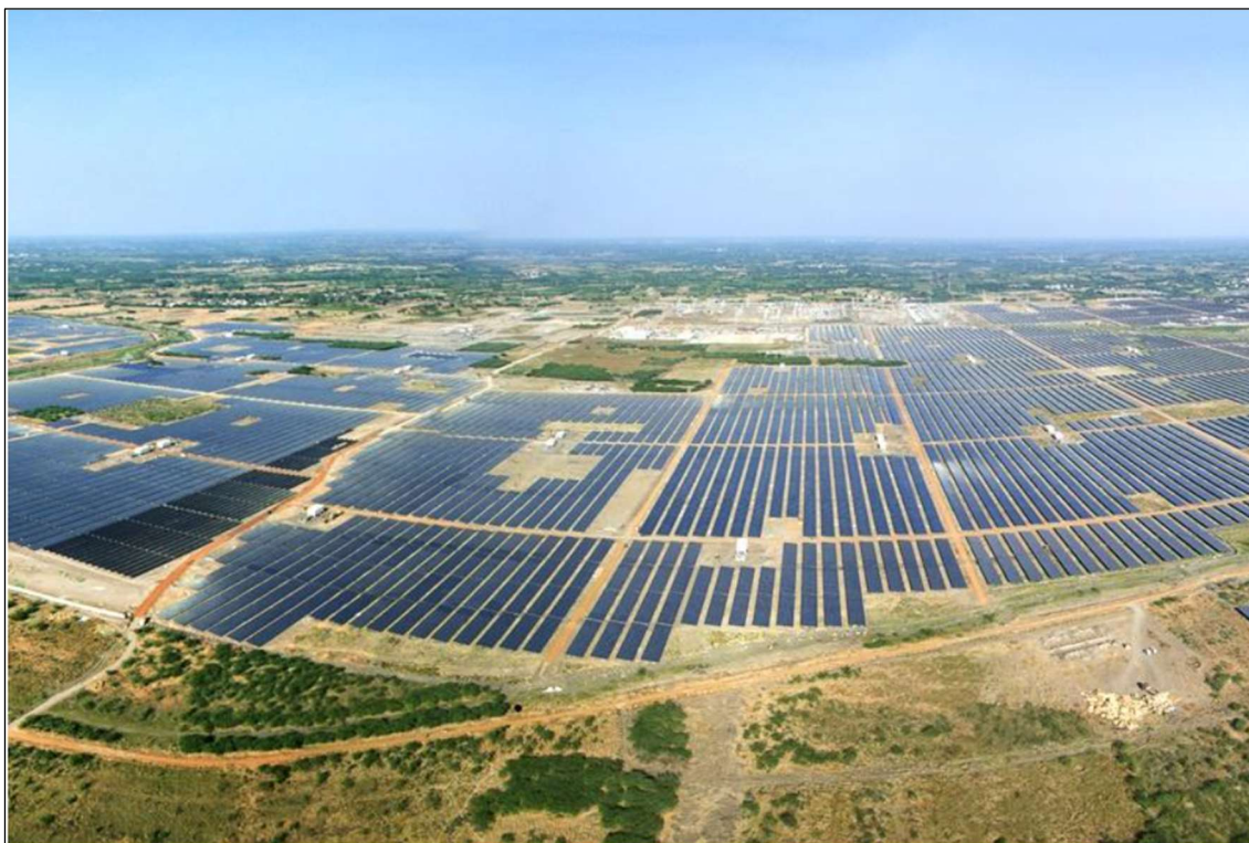
Figura 16 - Kamuthi Solar Power Project (Índia)
