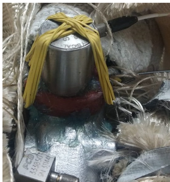
Figure 41 – AE set mounted on compressor housing
