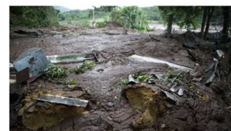
The mud covers the backyard of a house after a dam collapse near Brumadinho, Brazil, Saturday, Jan. 26, 2019. (Associated Press)
