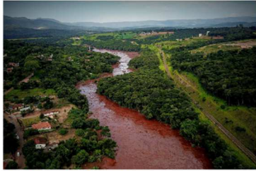
The dam at an open-pit mining complex is owned by the Brazilian iron ore mining company Vale. The disaster in Brejozão comes just over three years after a dam burst in the city of Mariana, 75 miles away, resulting in 19 deaths. (AP Photo/Chris Wedel)
