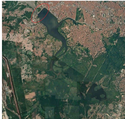
(c) Baganca dam location (circled in red).
