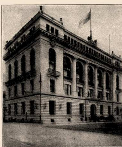
THE FINEST OFFICE BUILDING IN MEXICO THE BUILDING OF THE MUTUAL LIFE INSURANCE COMPANY OF NEW YORK
