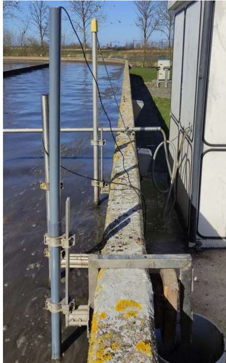
Figure 48 – US sensor (on the left) and optic sensor (TSS) in the carousel
