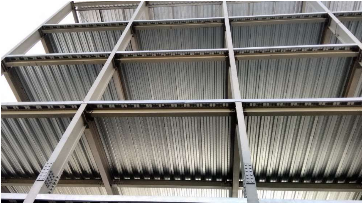
Figura 16 – Laje Steel Deck
