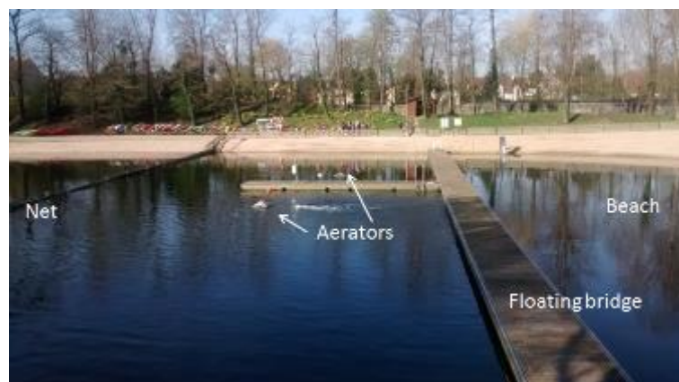
Figure 3.8 – Large beach and equipment installed. Photo: author, March 2017
