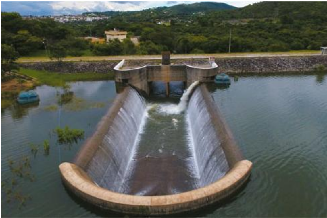
Figure 3.13 – Overflow in the spillway of Vargem das Flores reservoir, with pump installed in the right corner of the weir (31/01/2020)
