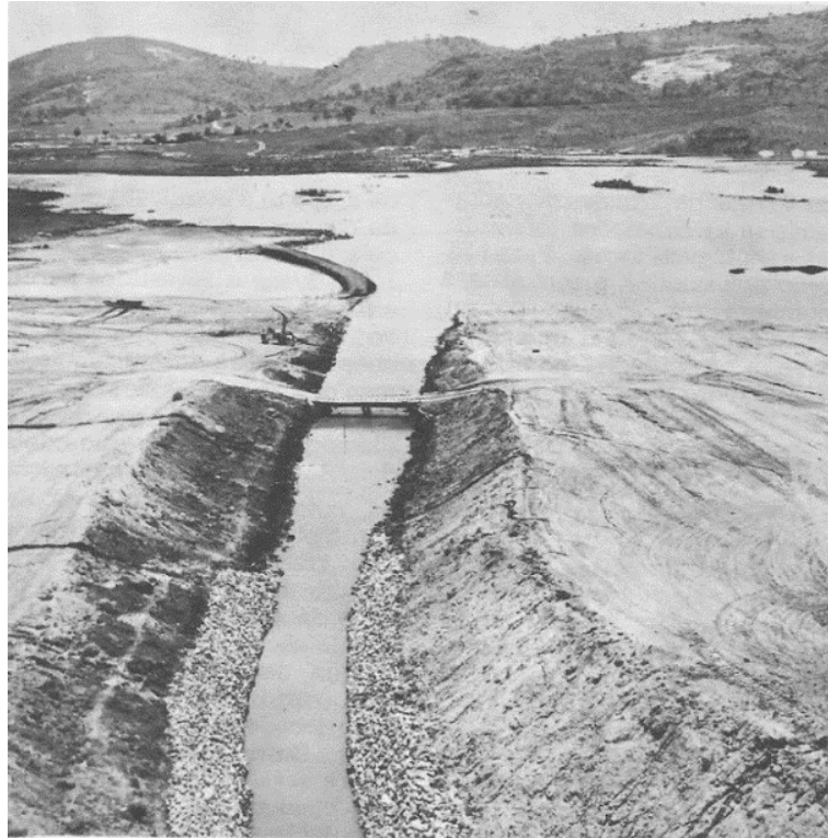
Figure 3.1 – Diversion channel of the Betim stream and the area that would be flooded by the reservoir (photo taken in 1968-1972)
