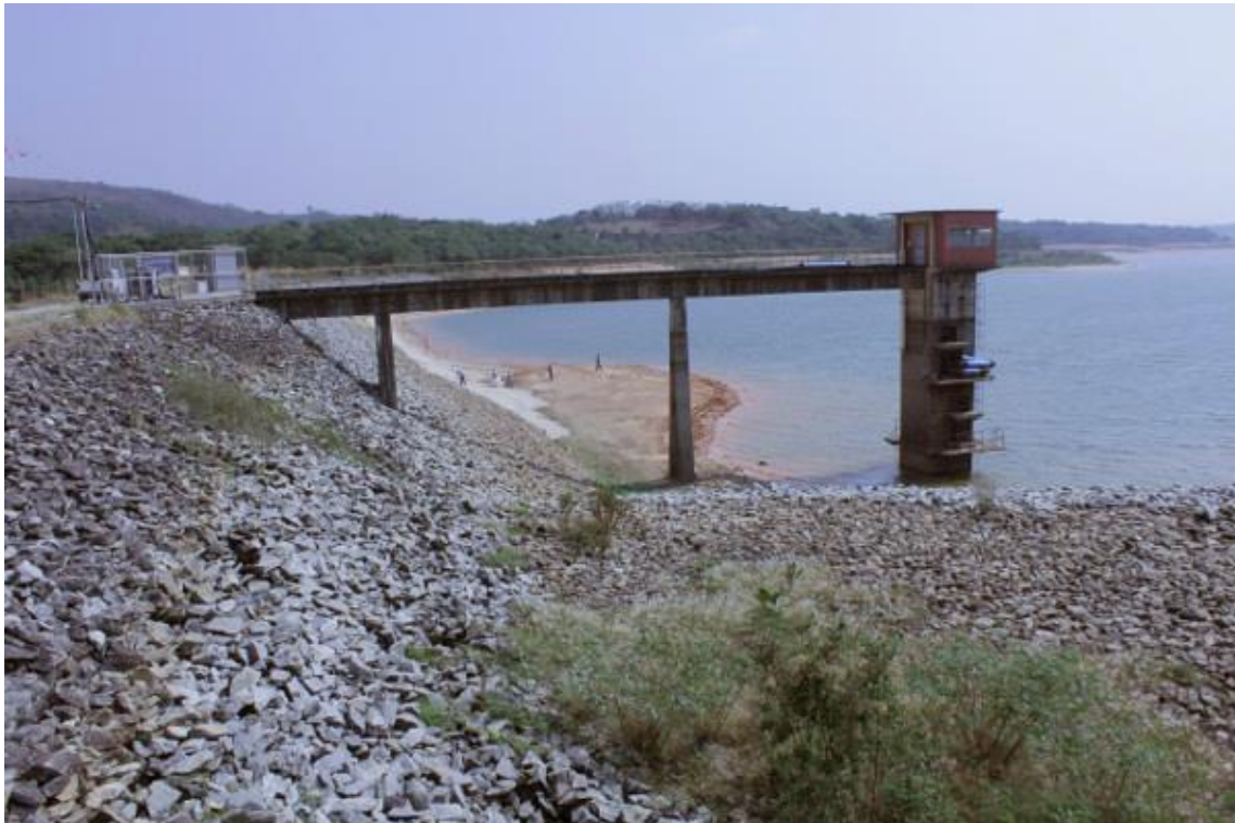
Figure 3.11 – Water intake in Vargem das Flores reservoir in the period of severe drought, 20% full reservoir (end of 2015)
