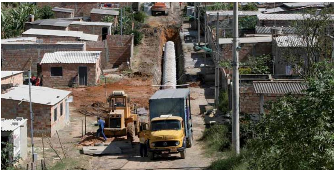
Figure 3.5 – Construction of sewage network in the region of Nova Contagem (2010)
