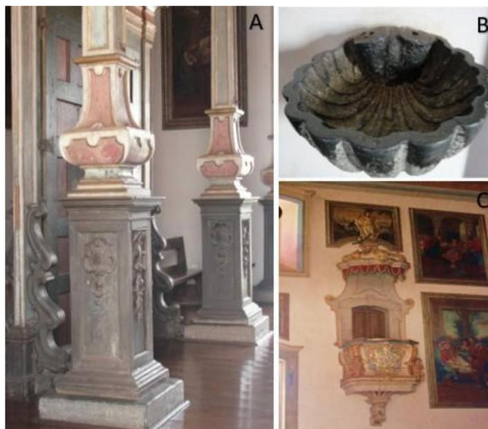
**Figure 4:** In the internal portion of the church, soapstone was the only stone material used. It is present in the staircase and outline of the high altar, besides the columns (A), bases, sinks (B), pulpits (C), arch, eaves, oculus, windows, doors and part of the floor present at the entrance.
