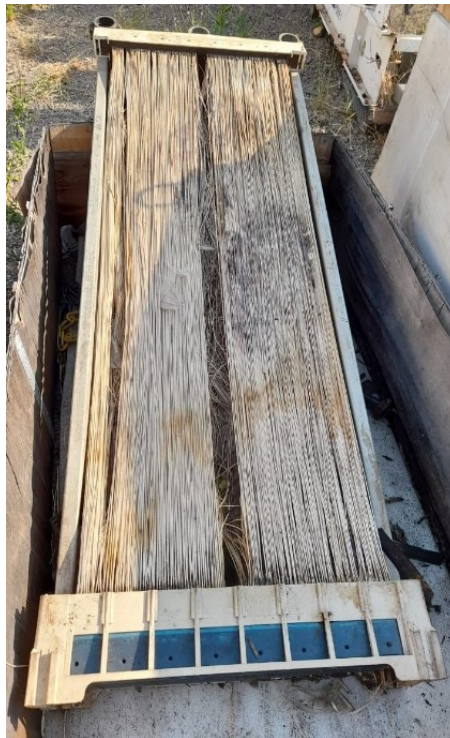
Figure 3.3 - Ultrafiltration (UF) membrane module discarded by the refinery
