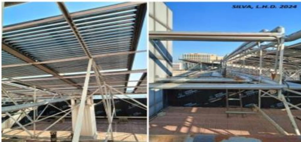
Figure 27: Solar system panel and pipes on Korea Building rooftop
