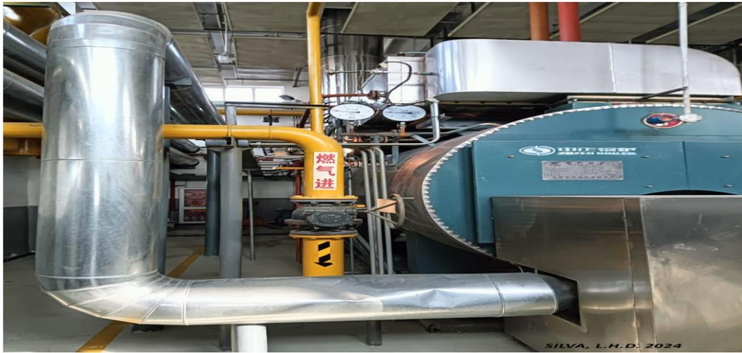
Figure 20: Boiler specifically designed to heat water for bathtubs and sink faucets
