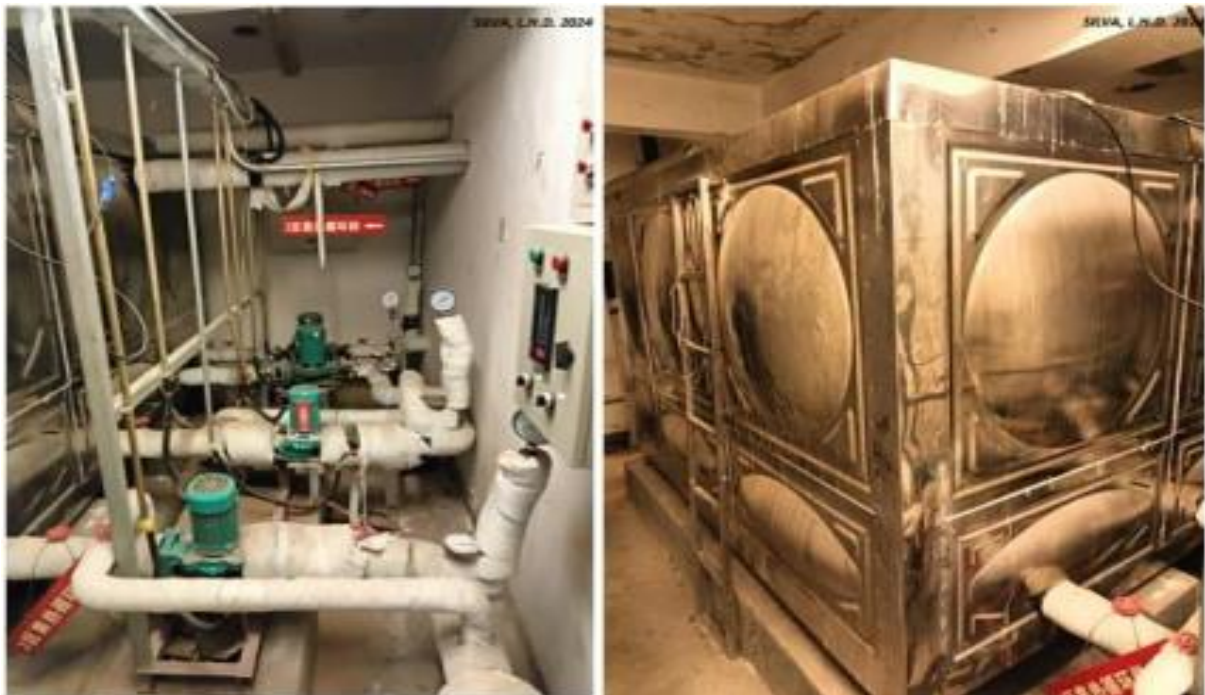
Figure 25: The pipes and the hot water tank on ISO rooftop
