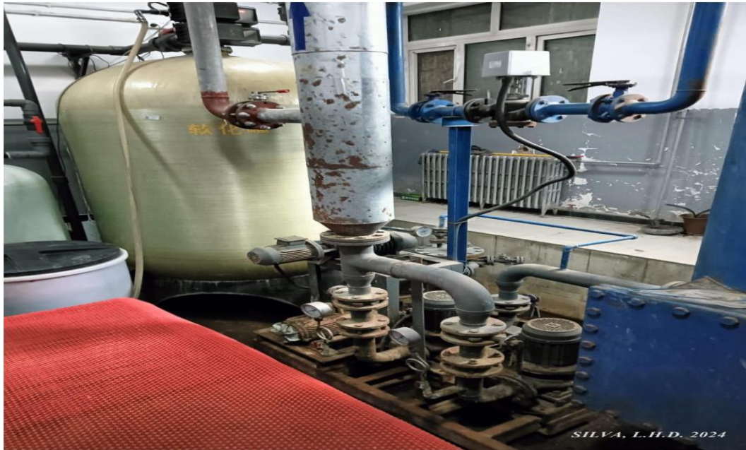
Figure 22: Components of the softening system
