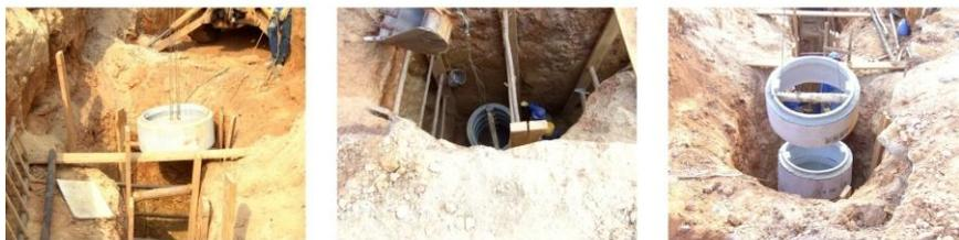
OS ANÉIS DESECEM APRUMADOS, POR GUINCHO OU RETROESCAVADEIRA, COM AUXÍLIO DE UMA ESTRONCA COLOCADA NA BOLSA INTERNA.
