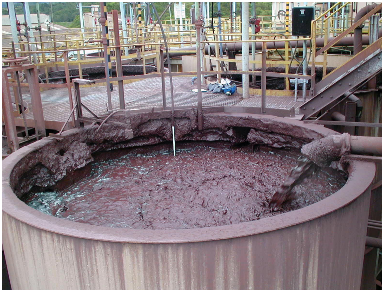
Figure 4.9 - Pre-lime Pachuca Tank at the Calcine Leaching Circuit
