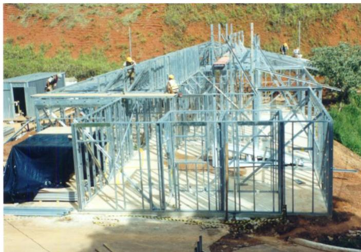
FIGURA 2.4 – Sistema Light Steel Framing
