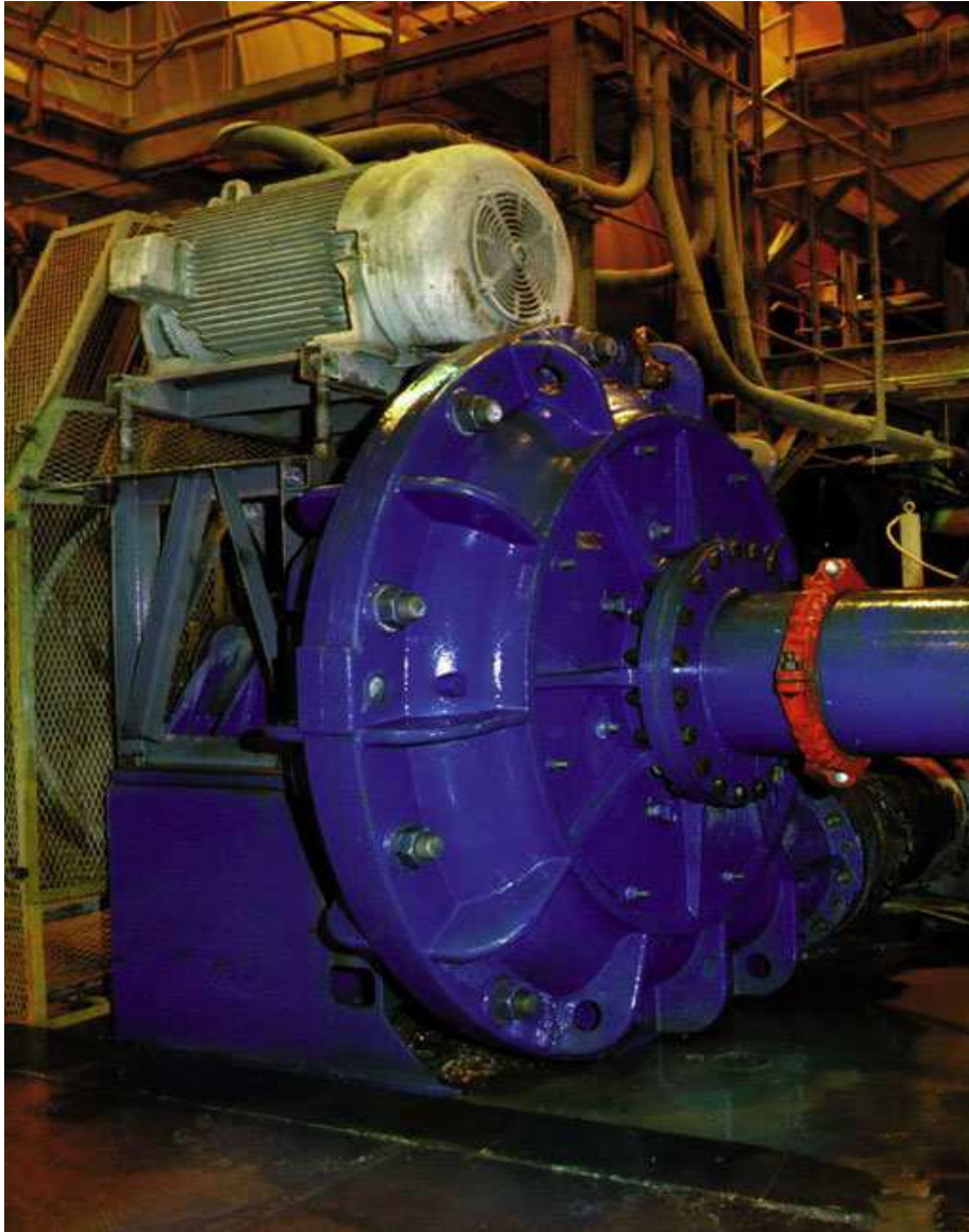
ASH PUMP 350 MCH pump. Ball Mill discharge application. Rubber lined casing, hard-metal impeller. Duty Q=1590 \text{ m}^3/\text{h} , H_m=14 \text{ m} , C_w=75\% . Drive: 225 kW, 1200 r/min motor and V-belts.
