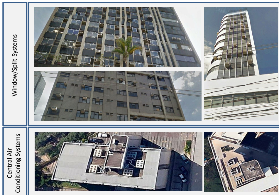
Figure 35 – Example of facade and roof images used to identify air conditioning systems
