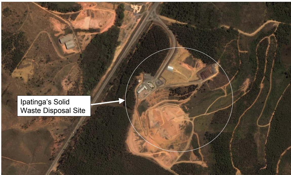
Satellite Photograph of Ipatinga's Municipal Solid Waste Disposal Site
