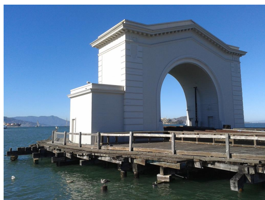
(a) Normal (original picture, no filter applied)
