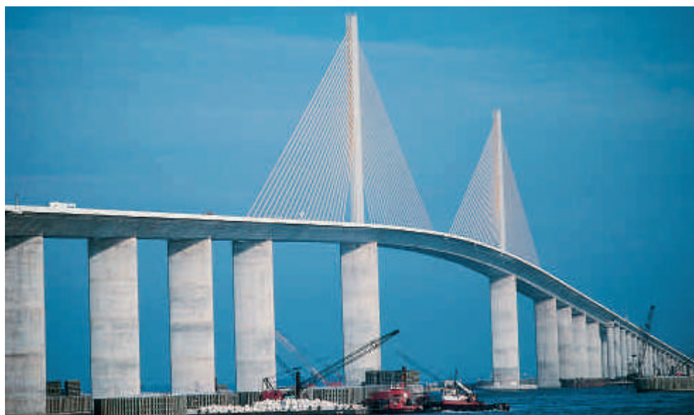
FIGURA 1.8 – Sunshine Skyway – Tampa-St Petersburg-FL-USA
