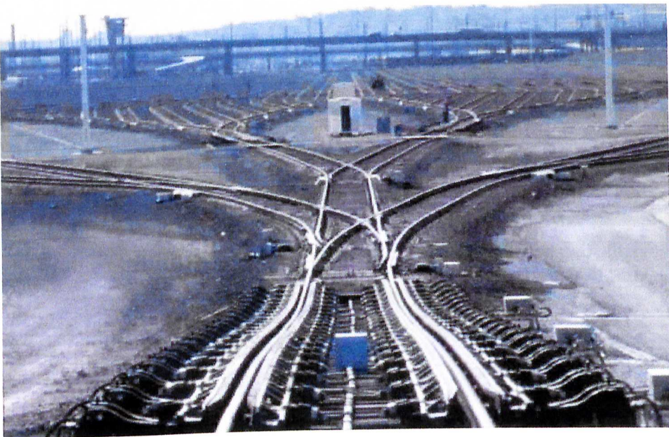
Figura 1.1 – Hump Yard da Burlington Northern Santa Fe's (EUA)
