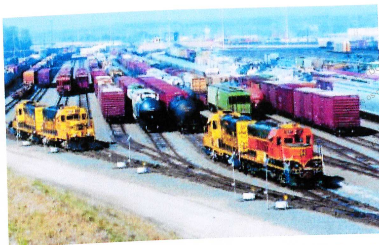
Figura 1.4 – Hump Yard da Burlington Northern Santa Fe's (EUA)
