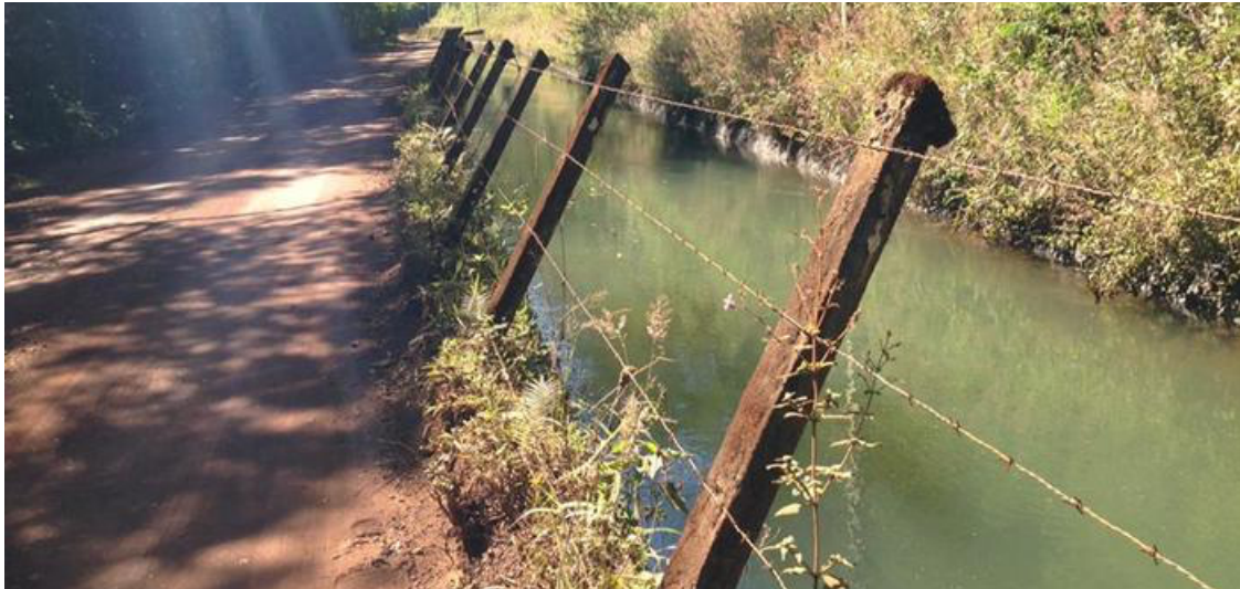
Figure 30: The Canal at Santo Antônio do Salto and the inadequate barrier provided by Novelis. Source: Ney (2015).
