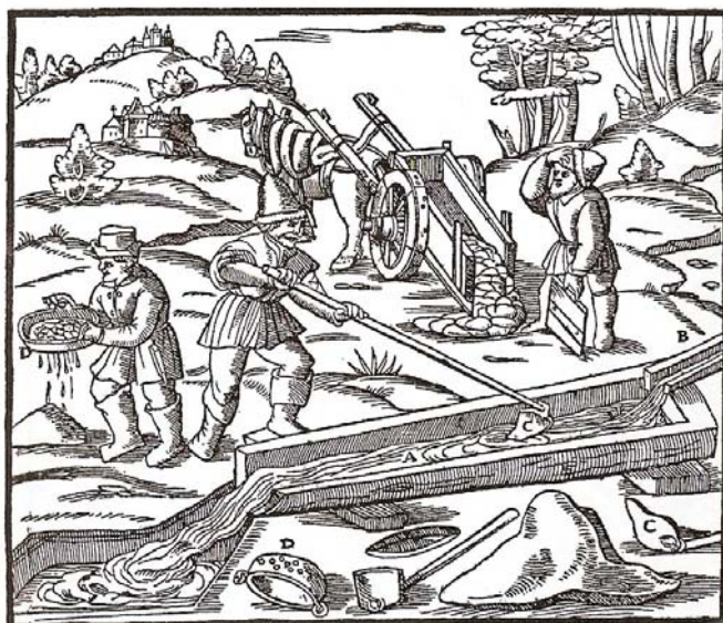
A—TROUGH. B—LAUNDER. C—HOE. D—SIEVE.
